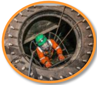
Tank & Vessel Cleaning
