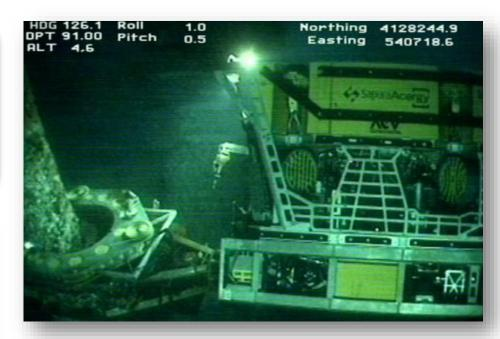
Client required contingency in the cutting technique, both external OD water abrasive and diamond wire cutting tools were engineered and utilised on the project
