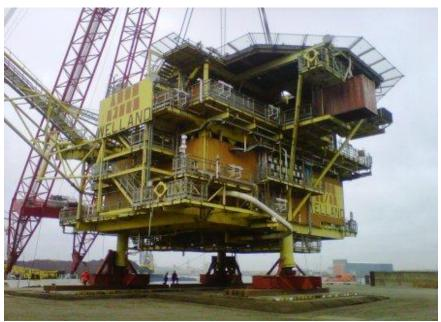
Topside and Jacket removed using a sheer leg crane and transported to Flushing Holland
