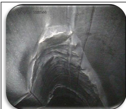
Image shows liners flexibility (coating over grout)
