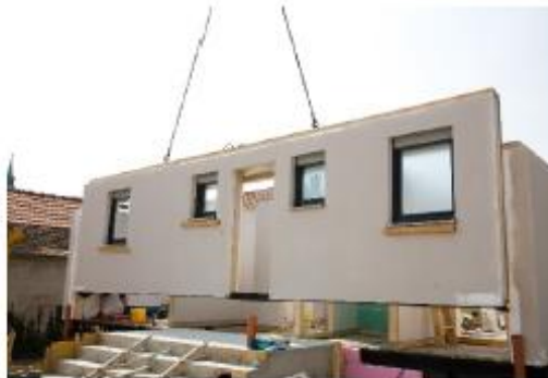
Transforming construction (up to £170m)
