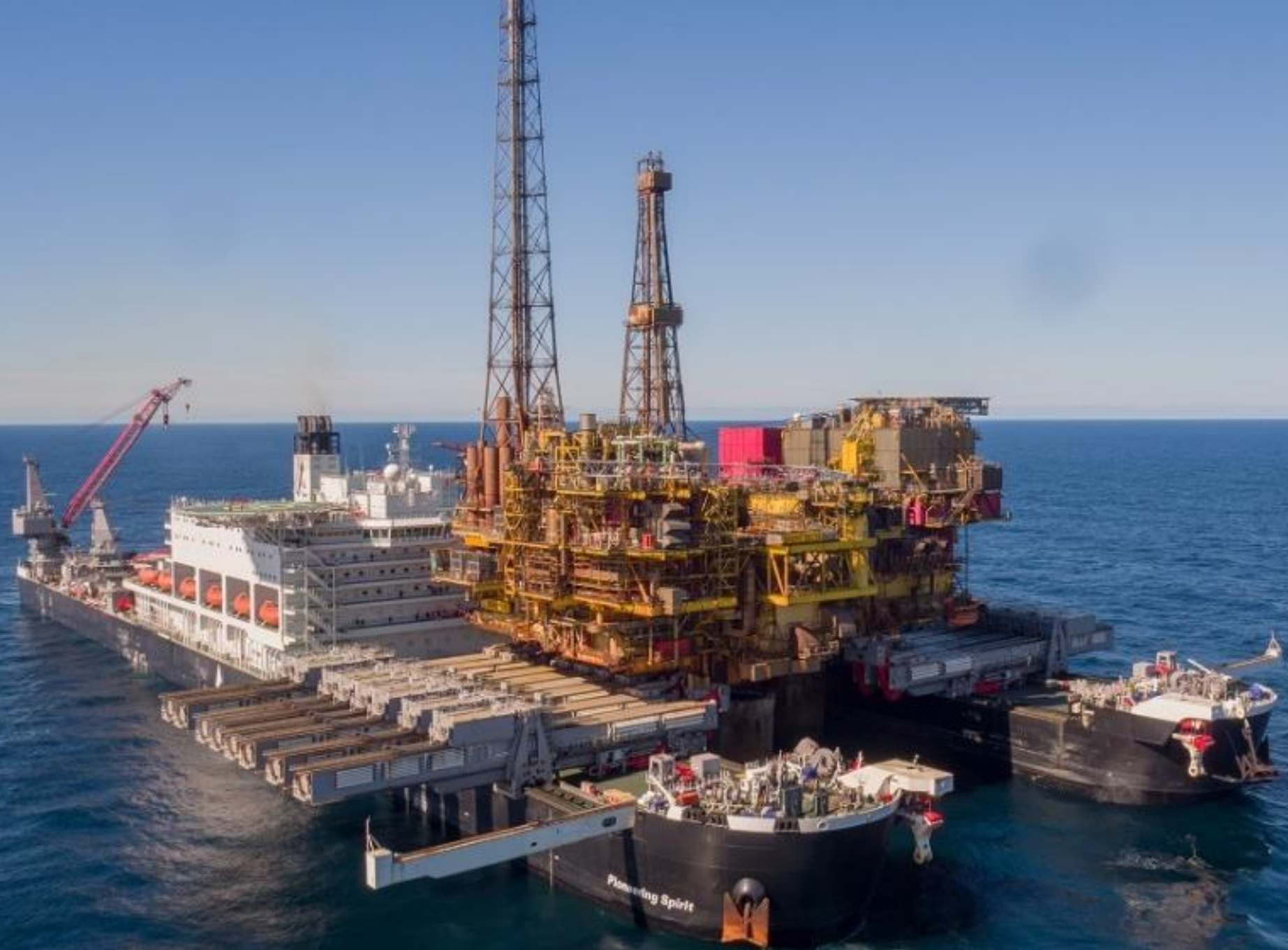
Single lift of Brent Delta topsides, April 2017
