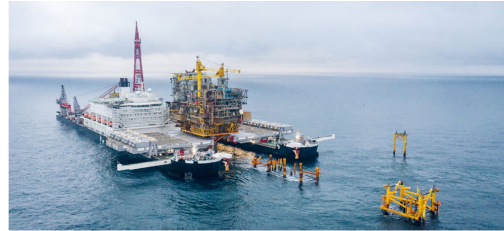
Tyra East A platform on its last journey
