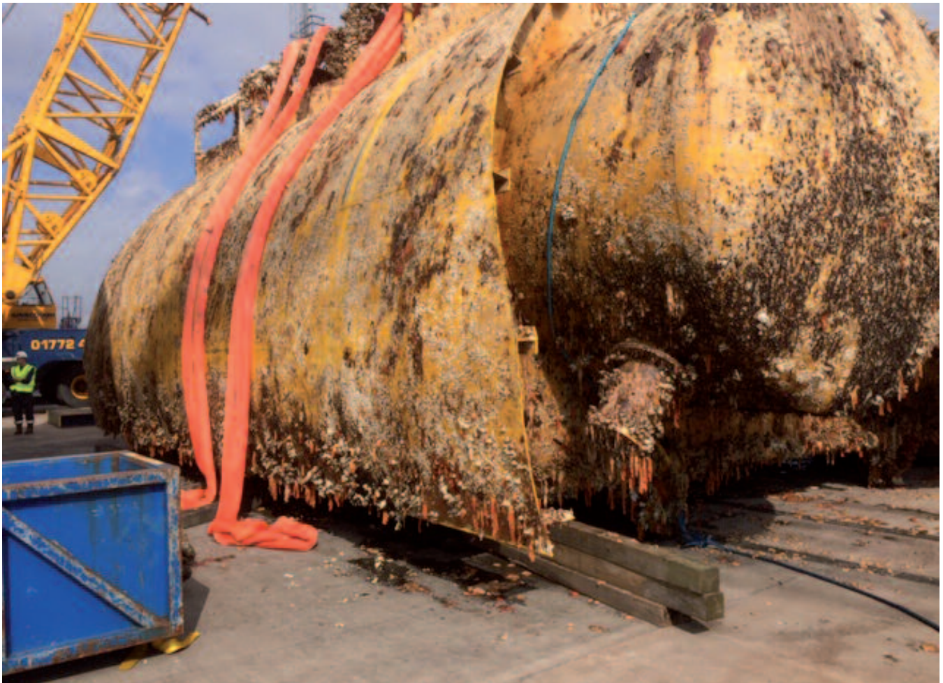
Figure 7: Management of marine growth a key issue at recycling and disposal yards. Source: Scotoil Services Limited (A Tradebe Company).
