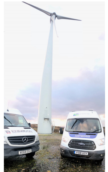
The wind turbine
