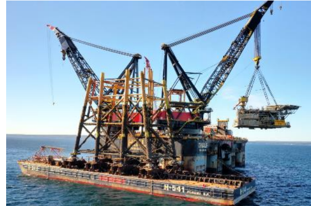
Sable Removal, Nova Scotia, June 2020
